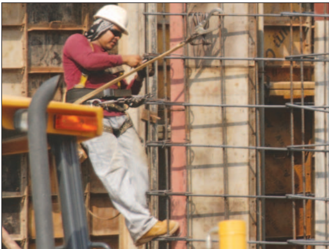
A construction worker continues renovations on W.G. Pearson Cafeteria.
